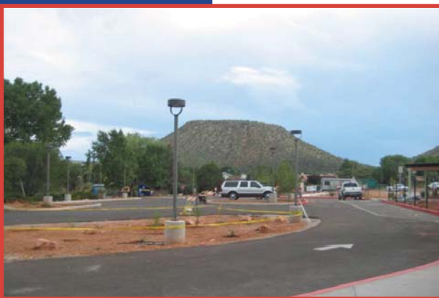
New Parking Lot
