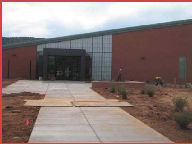
New Multi-Purpose Building
