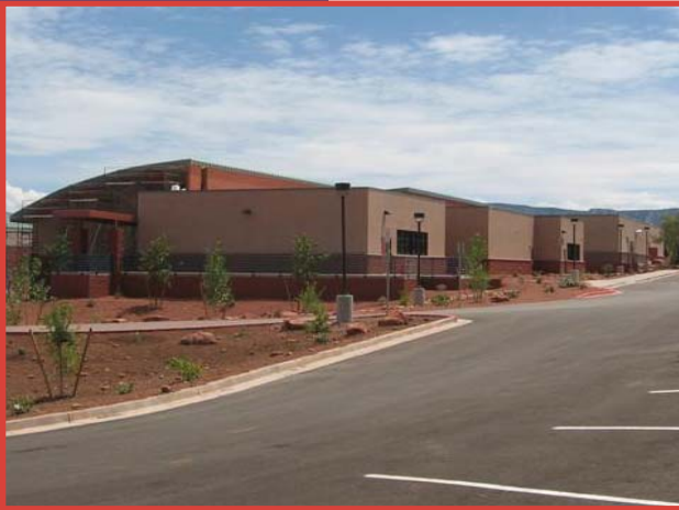
Additional Classroom Building
