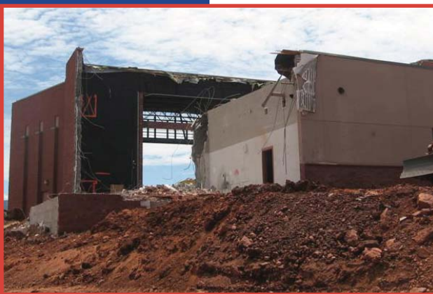
Demolition to Auditorium
